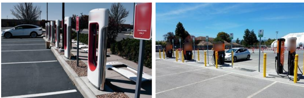
Figure 7: Installation of bollards to protect the charging stations
