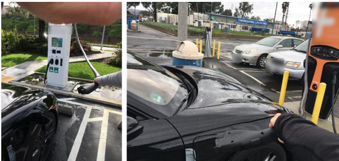
Figure 3: Insufficient cable length
